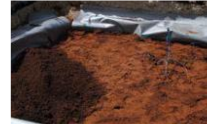
4. Add ArborRaft soil to top approx. 400mm of tree pit.
