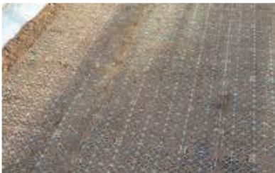
8. Backfill with ArborRaft Soil
