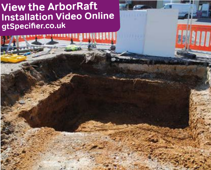
1. Excavate tree pit to include 500mm supporting shelf at the top of the tree pit.
