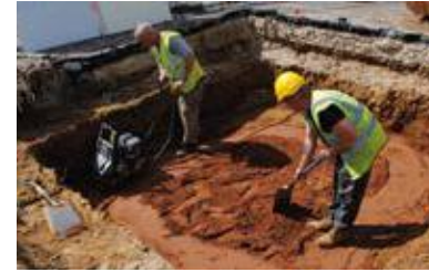
3. Install gt anchoring system and compact subsoil to architects specification.
