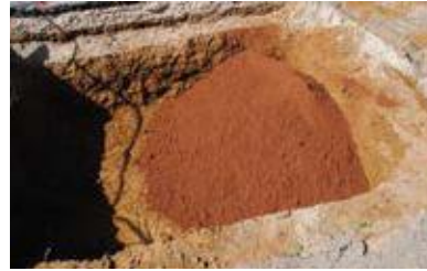
2. Backfill lower pit with approved subsoil, position tree or leave vacant for planting season.
