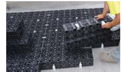
7. ArborRaft units simply lock together with connectors.
