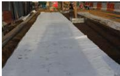
9. Cover with Arbortex 300 Membrane and finish to hard landscaping specification.
