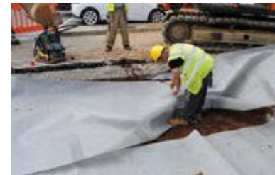
6. Cover with ArborRaft TRC30 Membrane.
