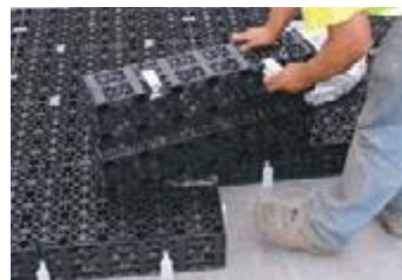
7. ArborRaft units simply lock together with connectors.
