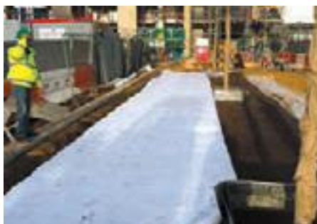
9. Cover with Arbortex 300 Membrane and finish to hard landscaping specification.
