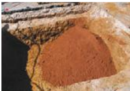
2. Backfill lower pit with approved subsoil, position tree or leave vacant for planting season.
