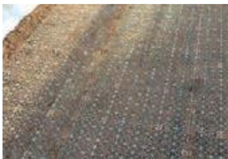
8. Backfill with ArborRaft Soil
