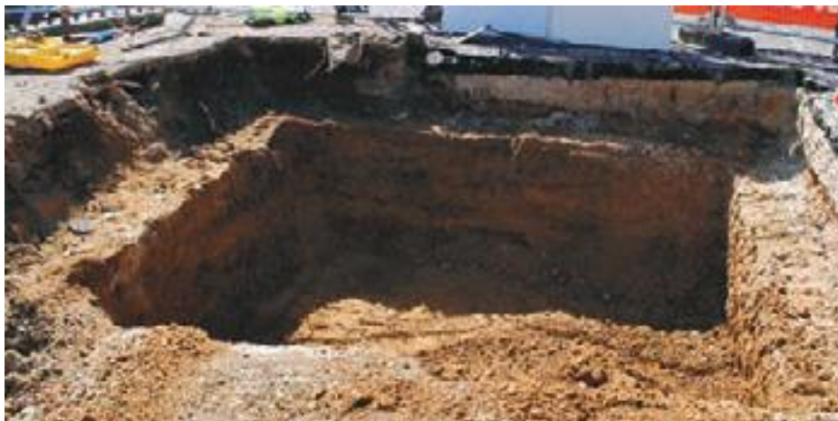
1. Excavate tree pit to include 500mm supporting shelf at the top of the tree pit.
