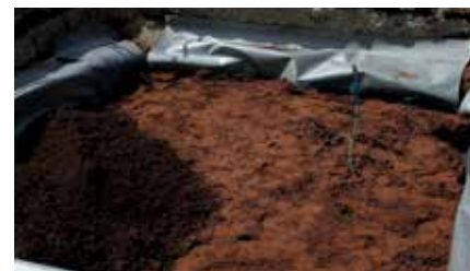
4. Add ArborRaft soil to top approx. 400mm of tree pit.
