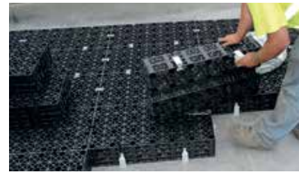
7. ArborRaft units simply lock together with connectors.
