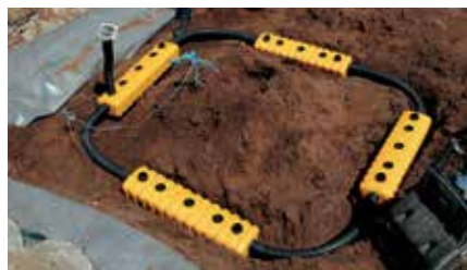
5. Install irrigation system.
