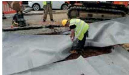
6. Cover with ArborRaft TRC30 Membrane.
