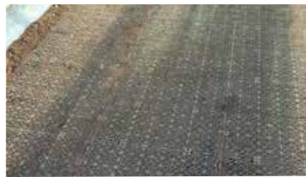
8. Backfill with ArborRaft Soil
