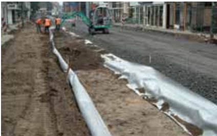
gtRootBarrier 325 installed on a high street
