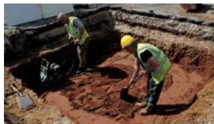
3. Compact subsoil to architects specification
