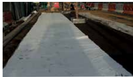
9. Cover with Arbortex 300 Membrane and finish to hard landscaping specification.
