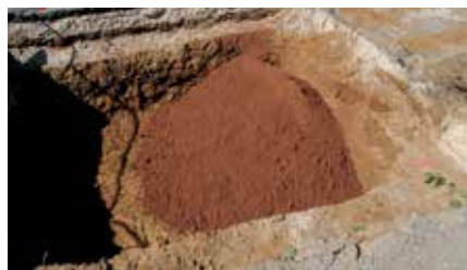
2. Backfill lower pit with approved subsoil, position tree or leave vacant for planting season.
